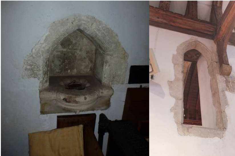
Photograph of Mediaeval piscina and rood screen doorway at the east end of the south aisle
