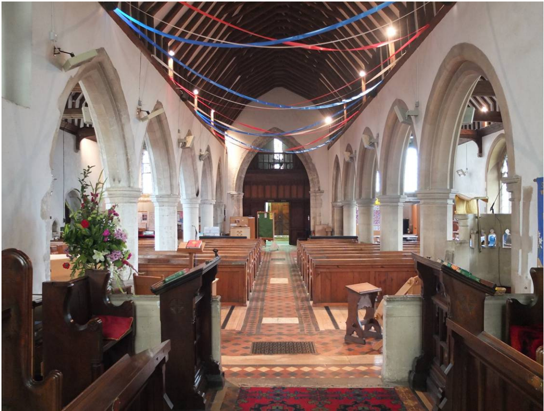
Photograph of the 13 th century tufa arcade on left and 19 th century copy on right
