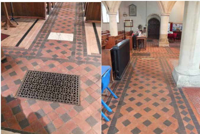
Red and black quarry tile passageways
